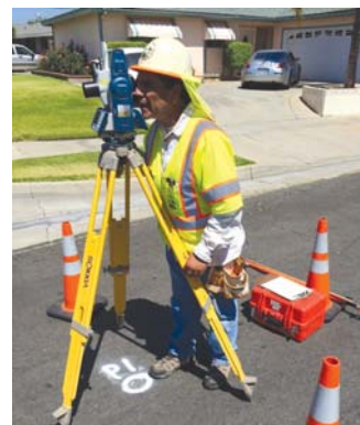
CAPE member Sam Quezada surveys a residential street in preparation for repaving.
